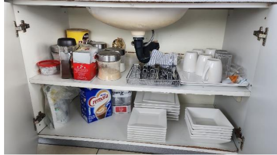
Figure 54. FARB sink and tap plumbing
