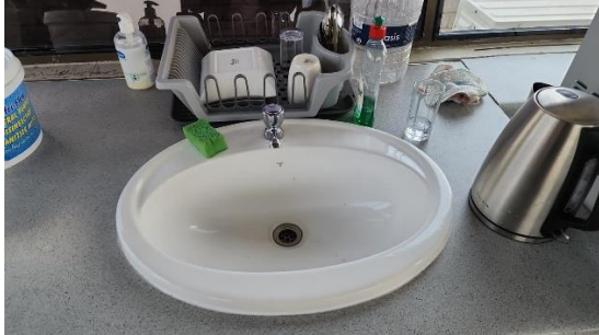
Figure 53. FARB Sink and tap.
