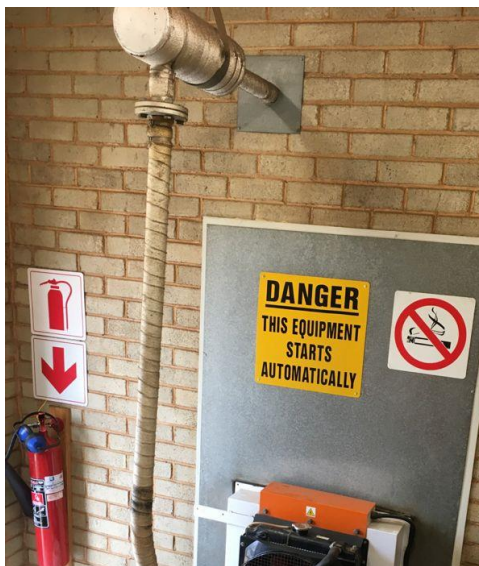
Figure 2: Exhaust pipe system
